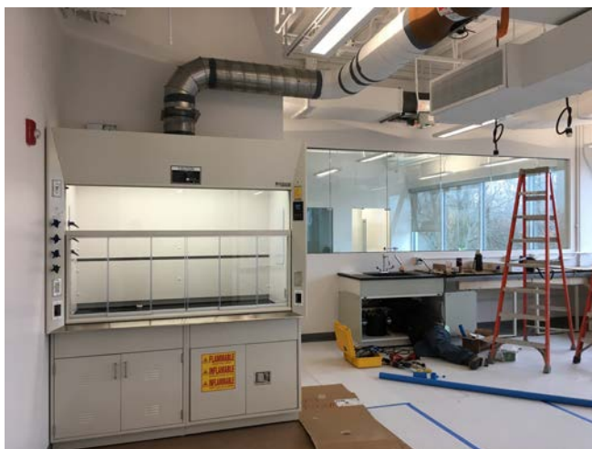
Battery Lab (construction photo)
